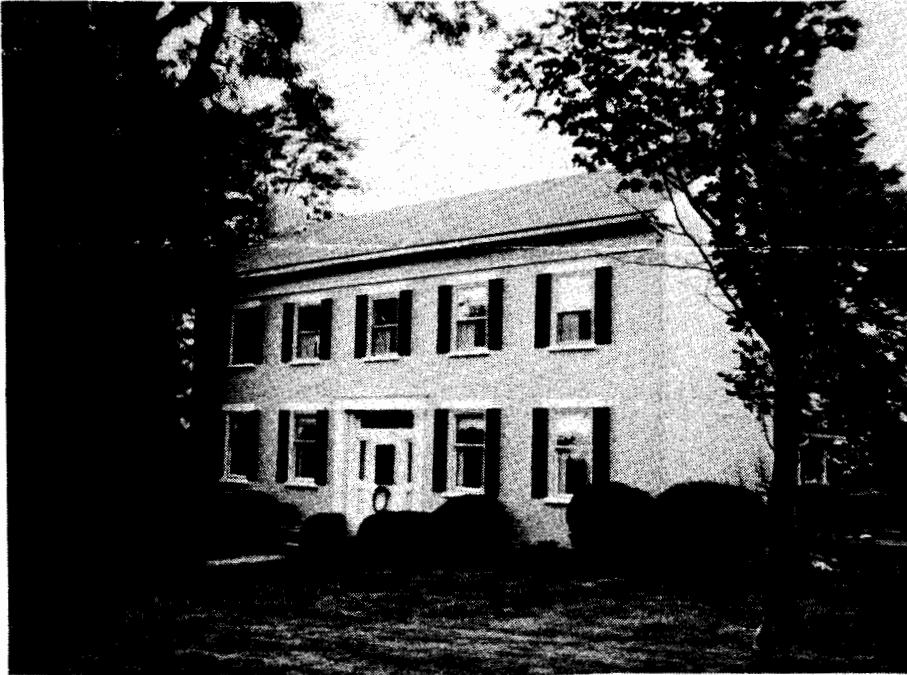
RICHARD RUE HOUSE now owned by John Sayre, one of the stops on the reunion bus tour.
